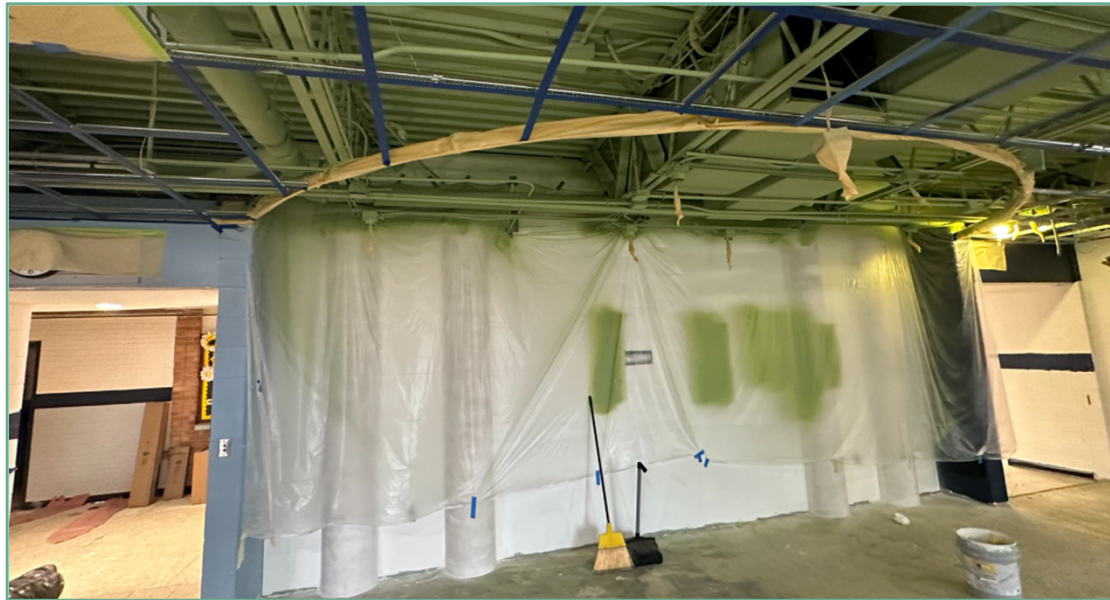
Gardens – Painting ongoing in media center
