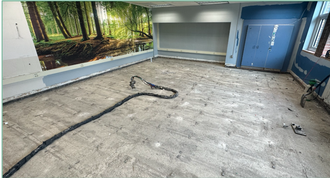
Morton – Slab stabilization complete
