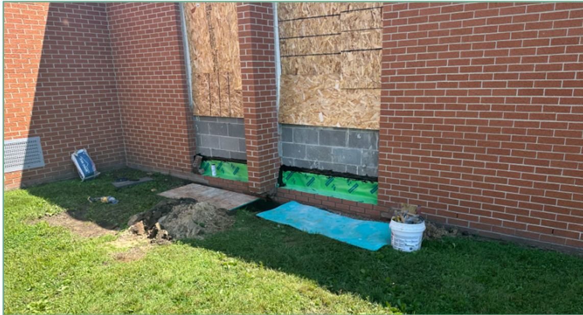
Gardens – Brick & sill repairs ongoing
