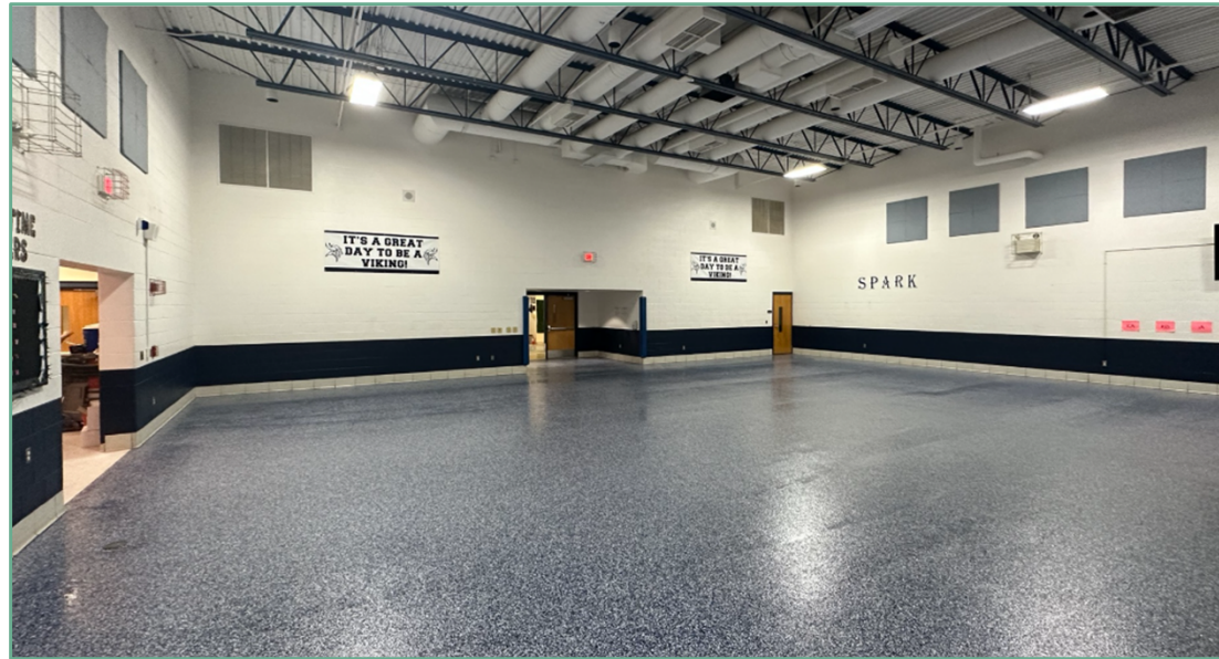
Morton – Epoxy flooring ongoing
