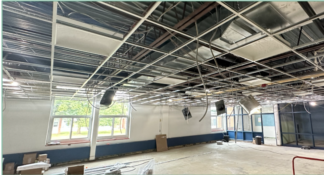
Gardens – New ceiling & lighting ongoing in media center
