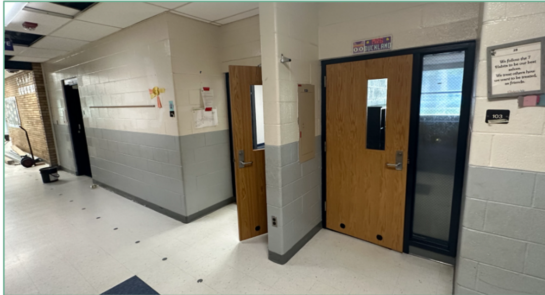
Washington – Painting door frames ongoing
