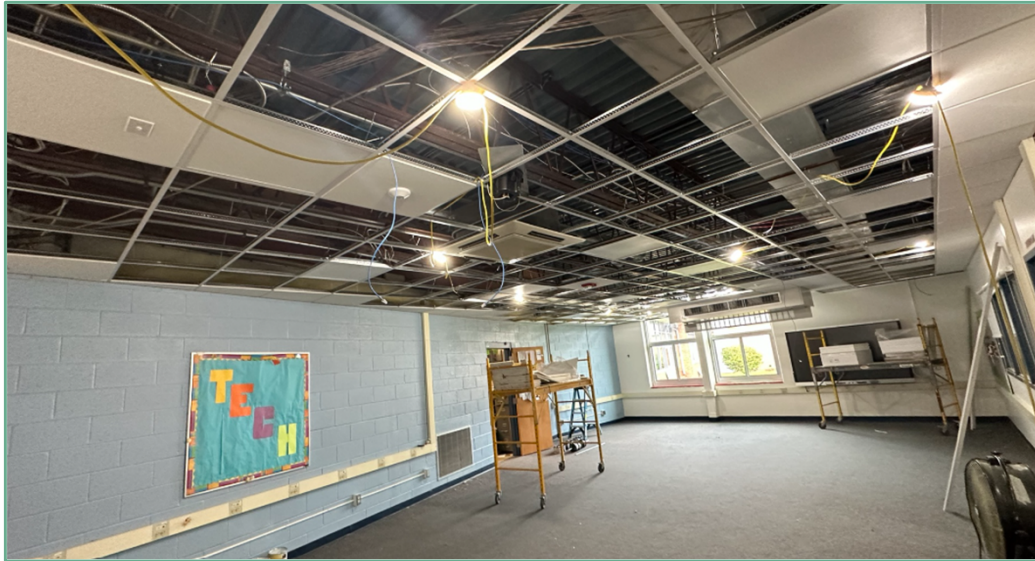
Gardens – New ceiling & lighting ongoing in tech room
