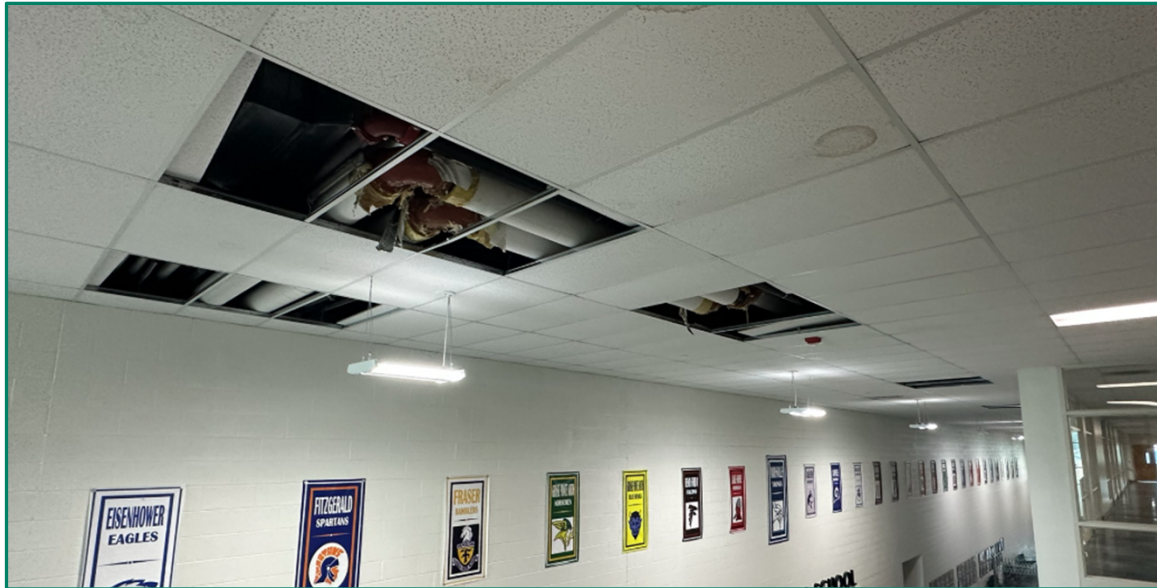
High School – Fitting change out – Complete
