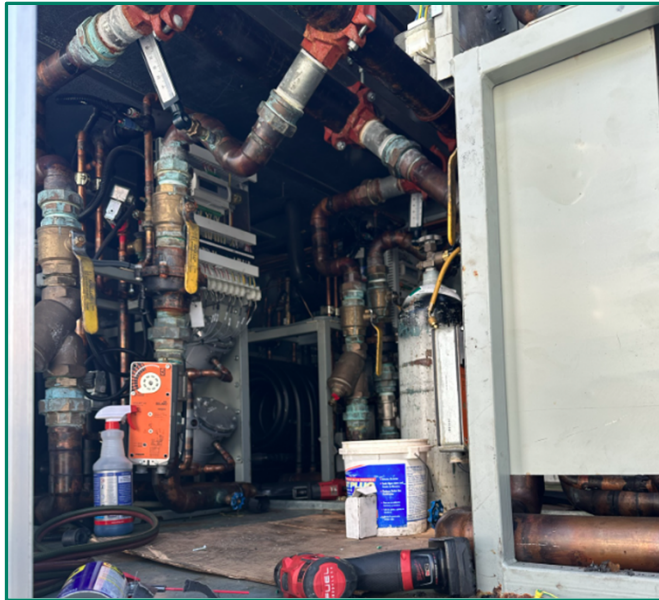
High School – Compressor replacements - Complete
